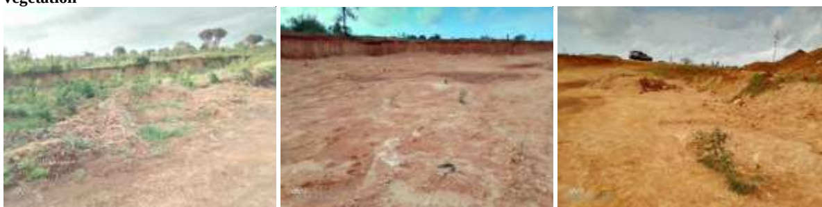
Plate 12: Un-rehabilitated material borrow site at Hindi Magogoni area Lamu County
