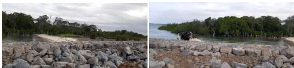
Plate 1: A section of on-going works at Lamu port at the causeway area which is adjacent to mangroves
