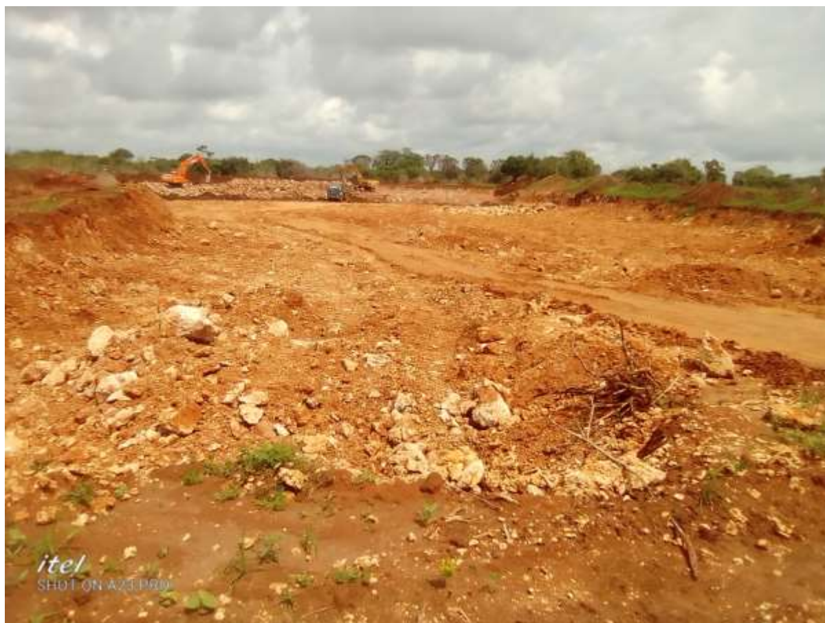
Plate 15: One of the active material borrow sites at Hindi Magogoni area of Lamu County
